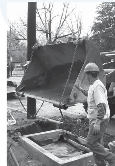
A tree-filter box is installed curb-side to filter pollutants from road runoff and to protect the health of a local stream.
