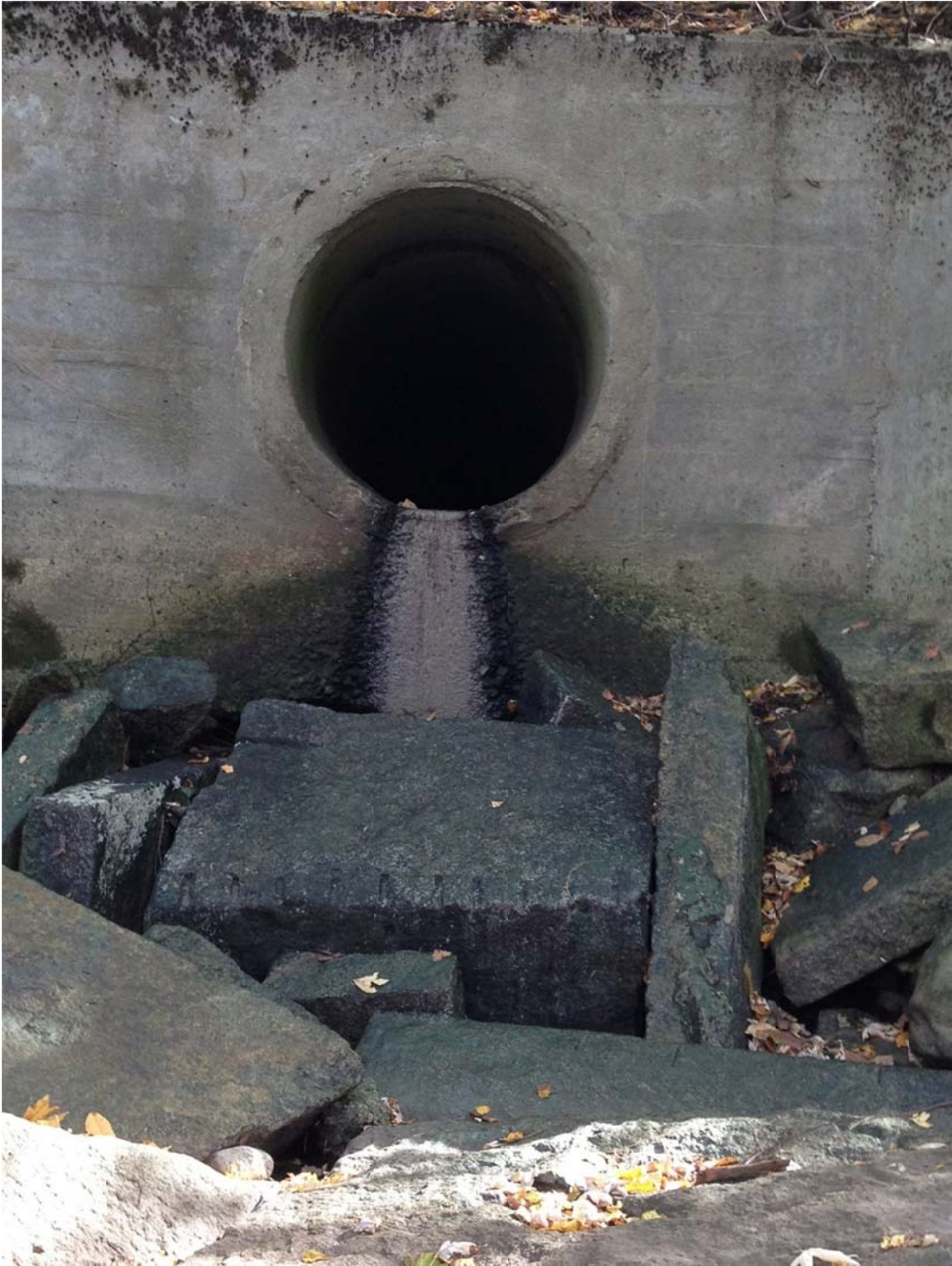
Figure 2: Image of outfall 4FSD0204 on 09/25/2012.
