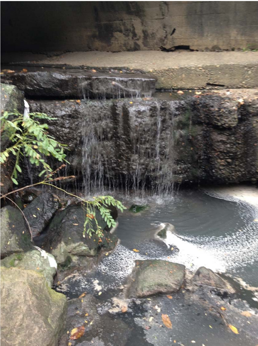
Figure 1: Image taken of outfall 7HSD0105 on 10/23/2012.
