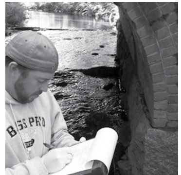
Inspecting and stormdrain outfall
