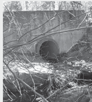
Lower Neponset River outfall pipe discharging water into the Neponset River.
